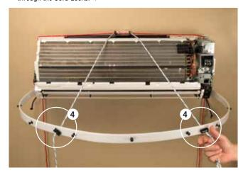
5. Attach the Funnel Bag to the frame by rolling it over the C-Band from the inside. Secure the mounting holes in the bag to the mounting studs along the C-Band. ▼
